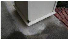
The lower sections of the front porch post show signs of decay and need repaired before further deterioration occurs.
