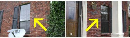
One or more window shutters were either damaged or found missing. Replace or repair as needed.
